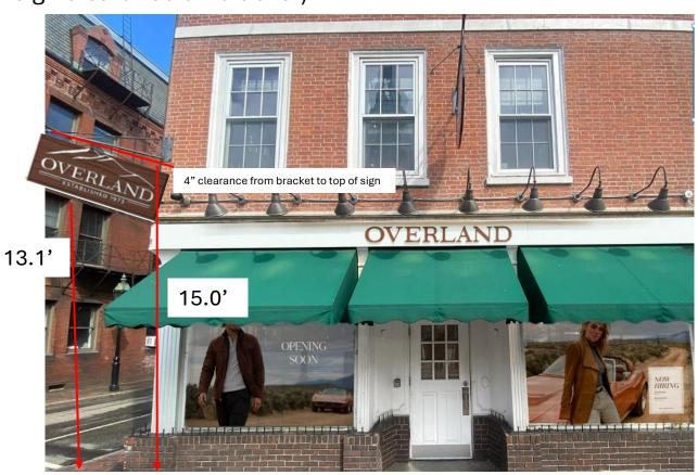
Sign 2 = 13.8' from sidewalk to sign bracket 11.9' from sidewalk to bottom of sign (including a 4" sign clearance off bracket).
